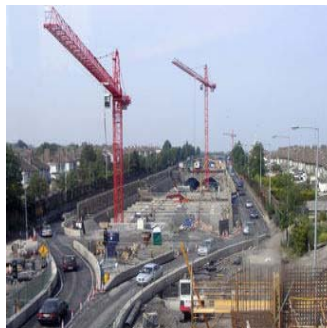
Inland entrance to Dublin Port Tunnel
